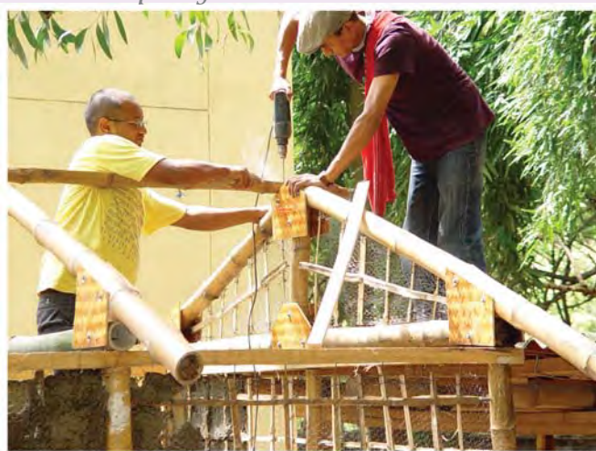
Mounting the trusses
