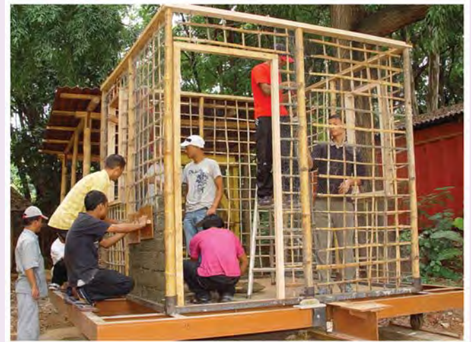
Infill wall construction
