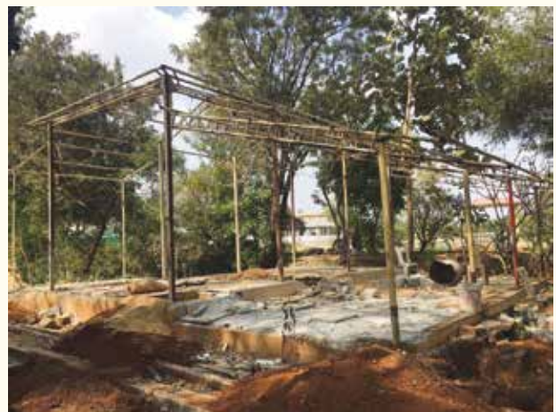
Site for construction inside Botanical Garden Campus
